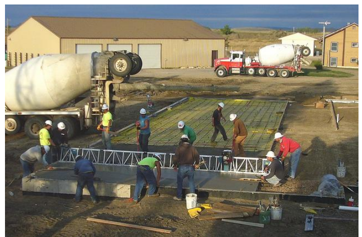
Figure 1: Slab on Grade Foundation. Credit flickr user US Forest Service
